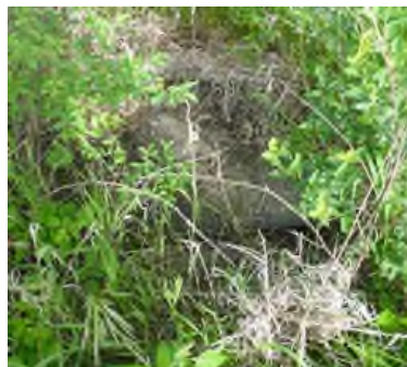
Holes and pits obscured by growth
