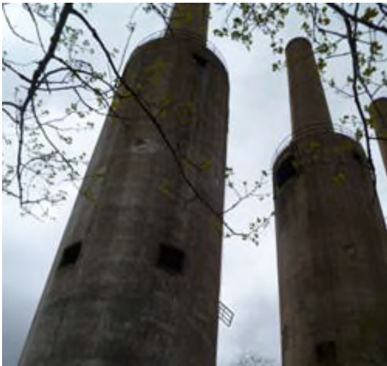
Fall Hazard: Stacks have vertical cables that could invite climbers
