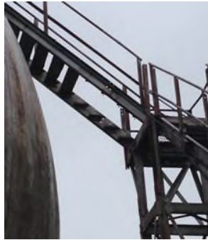
Fall Hazard: Deteriorated steps and supporting structures
