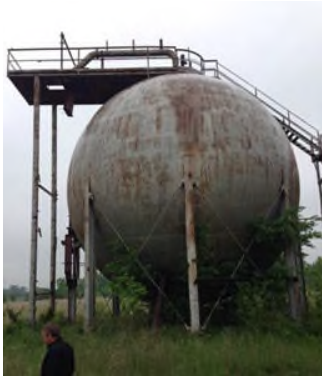
Fall Hazard: Deteriorated steps and supporting structures
